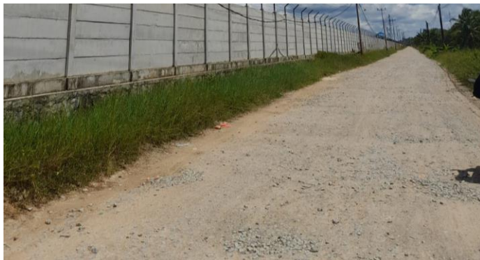
Figure 2. Road Access to Community Housing
